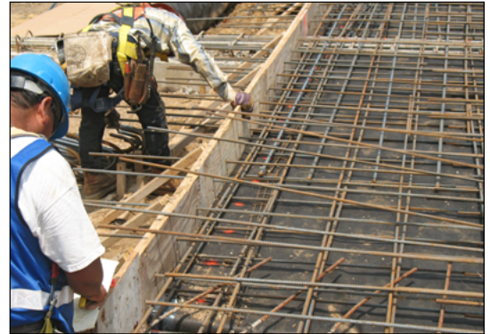
VBC-350 A Hospital Project, Dallas, TX
