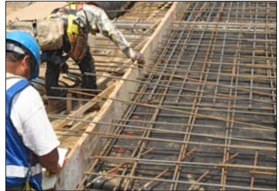
VBC-350 A Hospital Project, Dallas, TX
