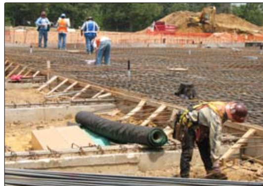
◀◀ A Hospital Project, Dallas, TX VBC-350 and void forms were used together in this project.
