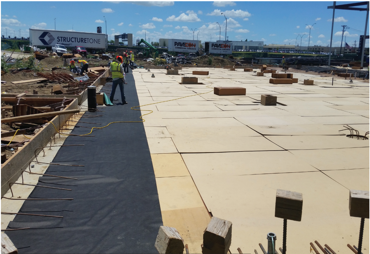
"VBC-350 Application with void forms in expansive soil area." (courtesy by VoidForm Products, LLC)
