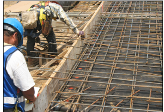
VBC-350 A Hospital Project, Dallas, TX
