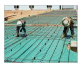
Our products are manufactured with a proprietary blend of polyolefin resins. This technology produces a product that will maintain a very low permeance & an extremely high puncture resistance throughout the life of the structure. Restricts migration of soil gases such as Radon & Methane.
