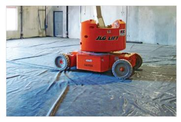
VBC-90 (18 mil) Floor Protection is recommended for both interior and exterior installations and can be easily removed at the completion of the project, revealing a clean dry floor that requires minimal clean up.
