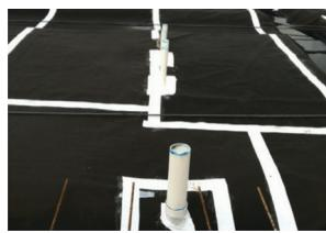
Our 7-mil White Bond Tape is made with a synthetic rubber compound which provides excellent bonding in low temperature applications. With easy-tear edges and no release paper, this polyethylene pressure sensitive tape is easy to use on the job site.
